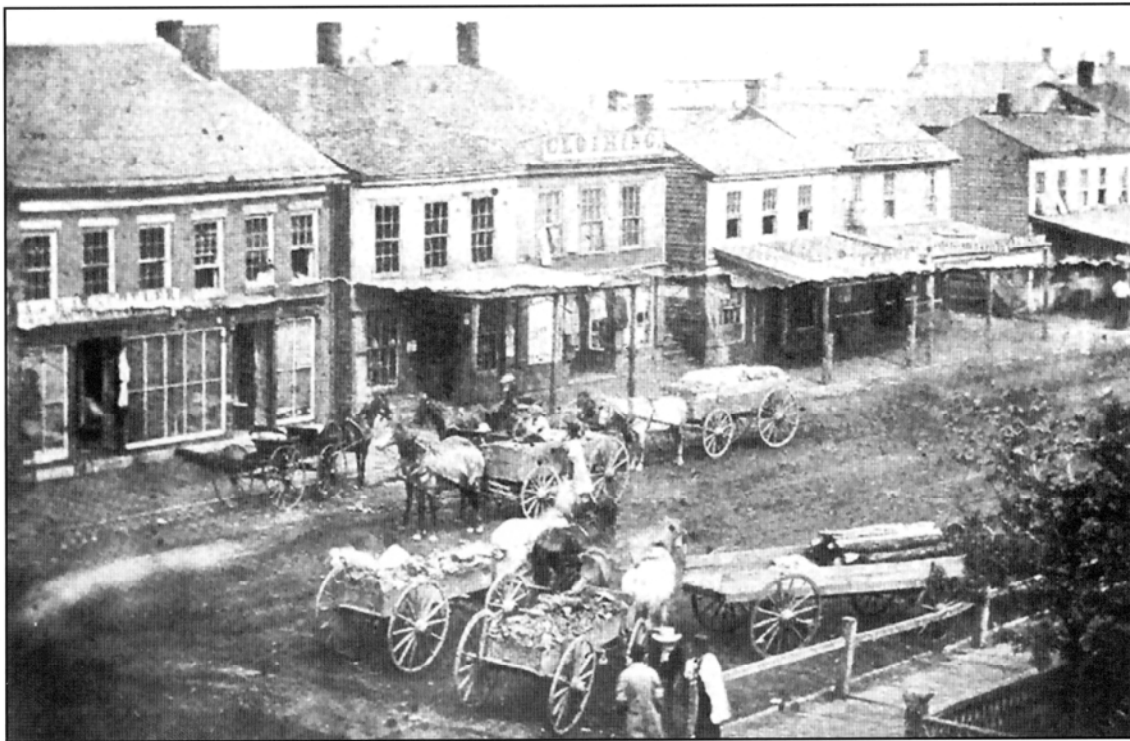
Image A3 – View of LaSalle Street across from Courthouse, ca 1860.
