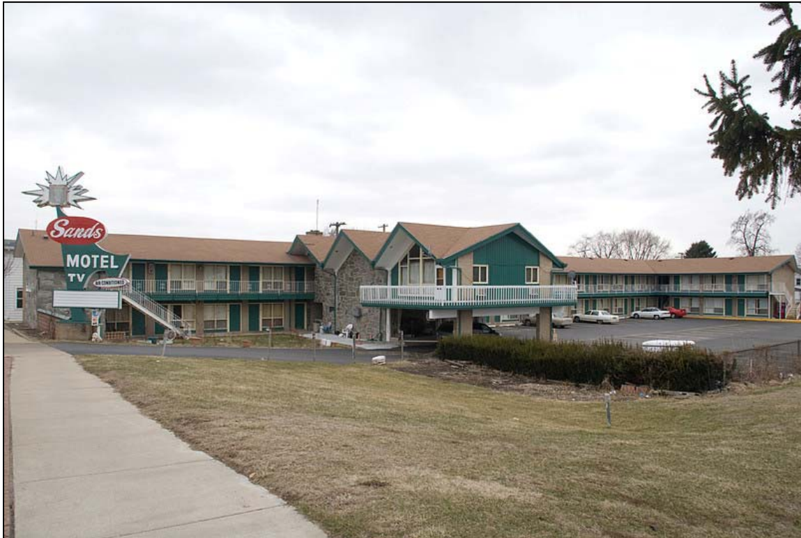
Photo 08: The Sands Motel
