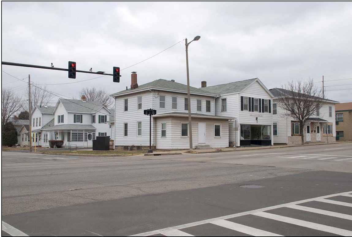
Photo14: Northwest corner of LaSalle and Superior Streets
