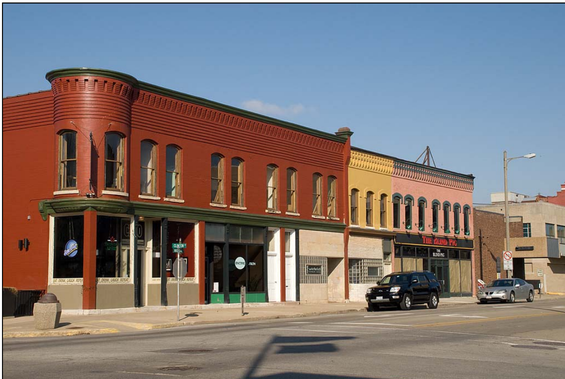
Photo 23: North side of the 200 block of West Madison street facing east
