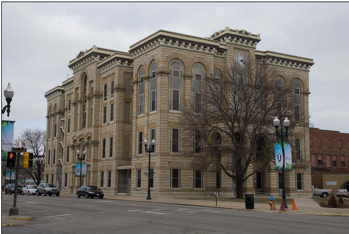
Photo 03: County Court House
