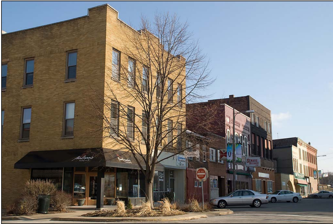
Photo 18: East side of Court Street facing south
