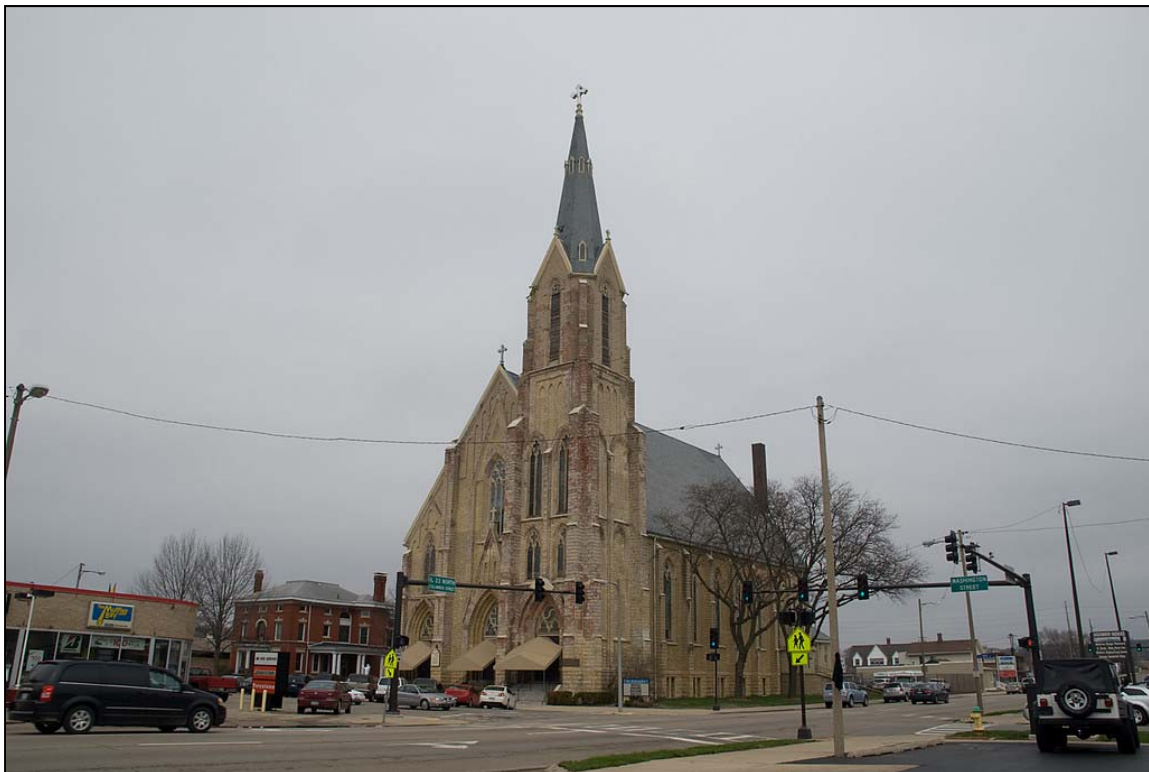
Photo 29: Northwest corner of Columbus and Lafayette Streets
