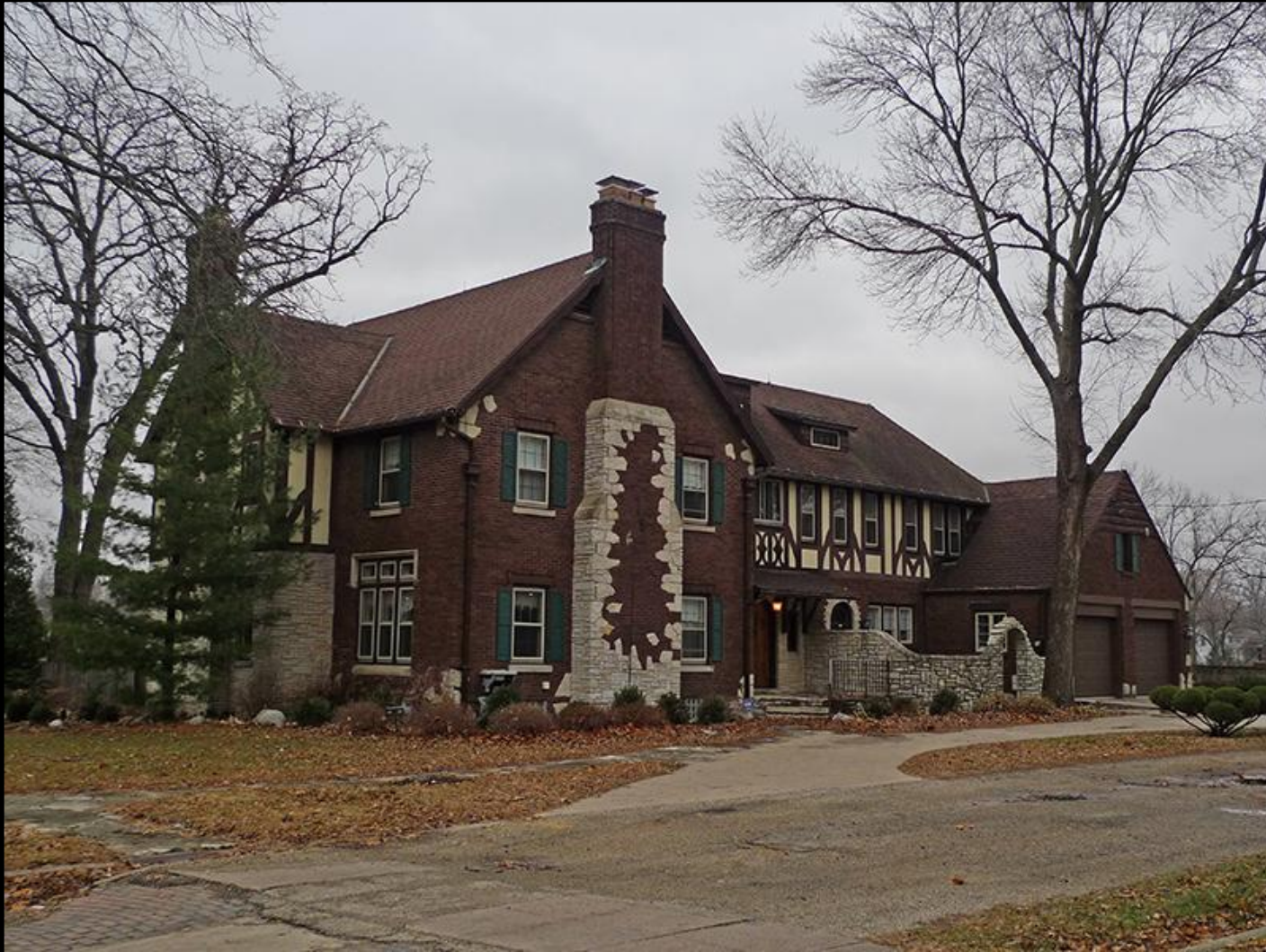
French-Wilson House (c. 1880, remodeled in 1929) 300 Pearl Street
