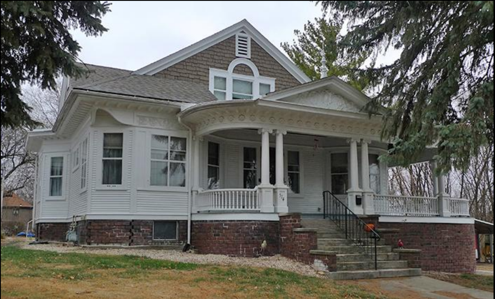
John J. Shanley House (1911-12) 514 Orleans Street
