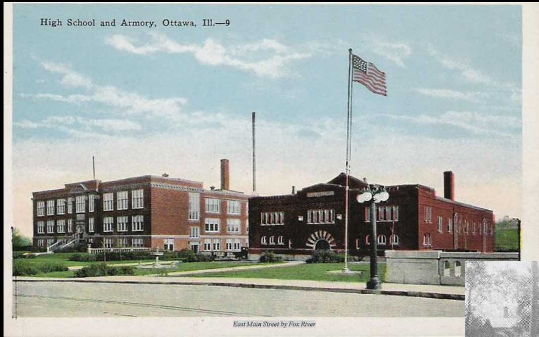
Armory (1912) & Ottawa Township High School (1916)
