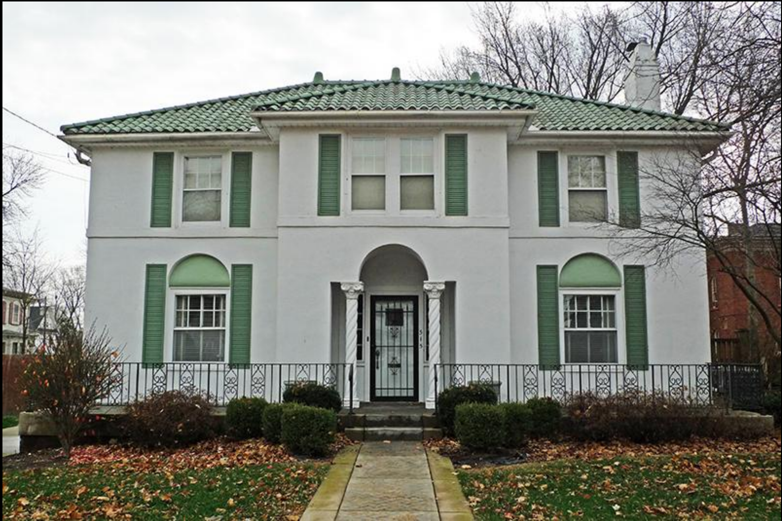
Guy Karr House (1926) 515 Pearl Street
