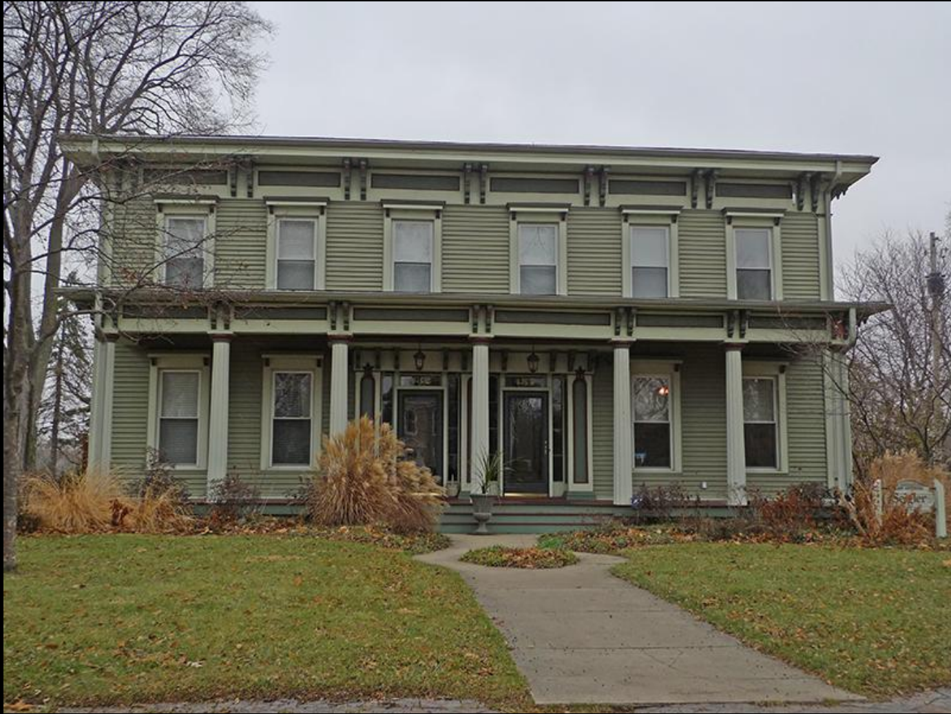
Reifsnyder House (c. 1860) 432-434 Pearl Street
