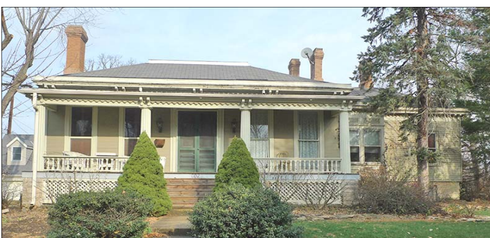
Florey-Cook House 602 Chapel Street
