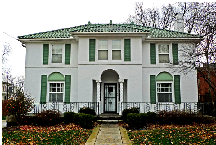
Guy Karr House 515 Pearl Street
