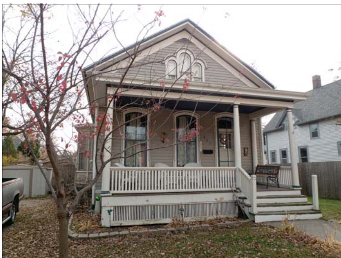
William Sinsel House 807 Chapel Street
