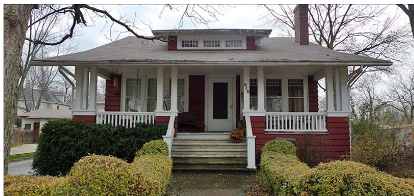
Milton Weiss House 815 Chapel Street
