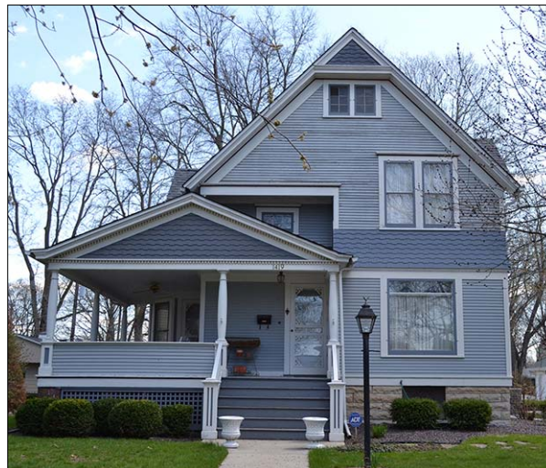
James M. Meekel House (c. 1900) 1419 Ottawa Avenue
