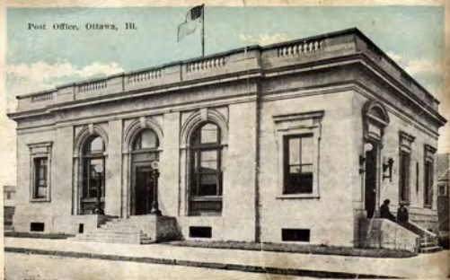
Ottawa Post Office - corner of Madison and Clinton
